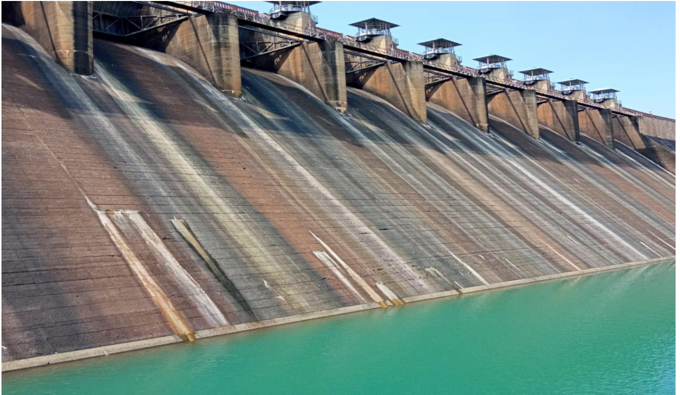
Picture of Ogee spillway
