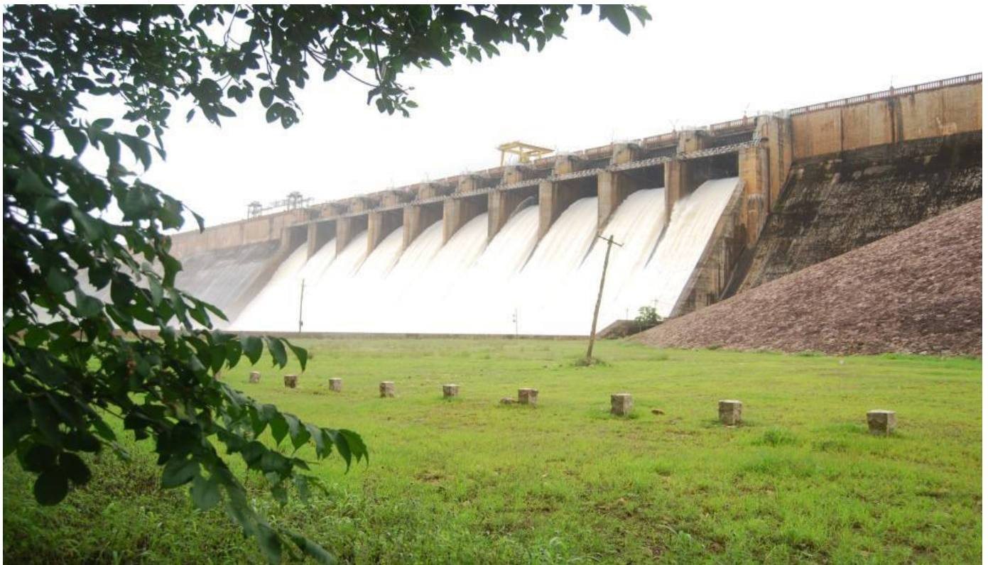
Picture of Dam spillway
